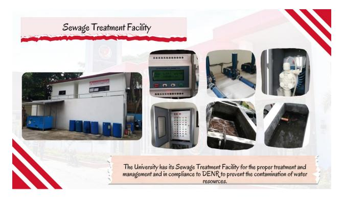
The STP is composed of equalization tank to stabilize the waste, aerobic digester tank to eliminate anaerobic conditions in the tank and prevent settling of suspended solids, two sequencing bioreactor tank that also serves as an equalization basin that tolerates peak flows or peak loads in the effluent that equalize them in the batch reactor. The chlorine tank is also included for the disinfection of treated water.
