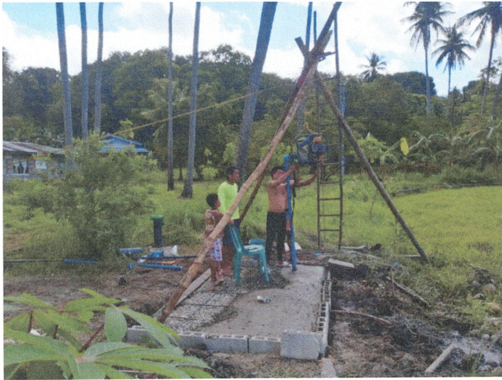
Figure 12. Construction of Deep Well
