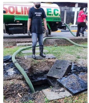
Siphoning of Septic Tank Located at the Side of SSC Building and CICS Building
