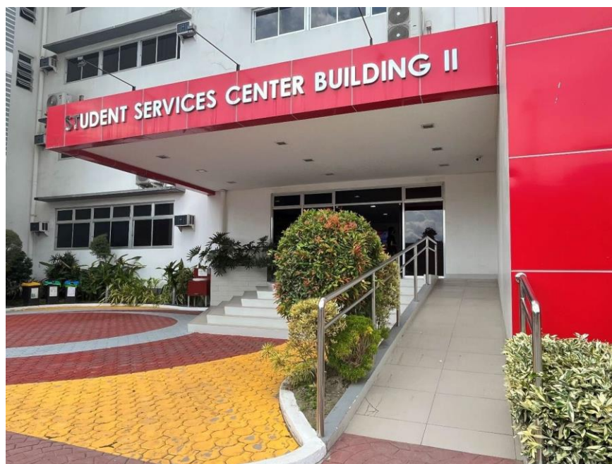
Ramp Passageway in the entrance of the Student Services Center Building II in BatStateU Pablo Borbon
