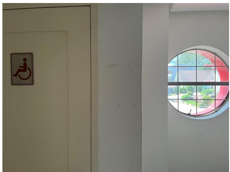
Restrooms constructed for persons with disabilities
