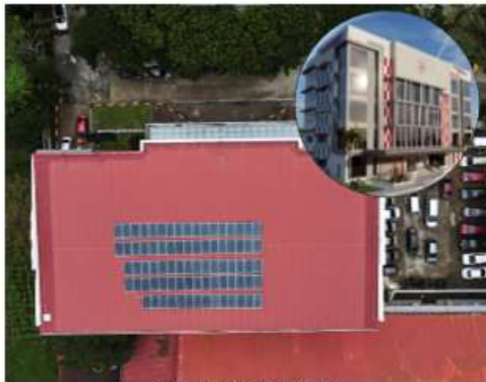
Five Storey STEER HUB Capacity 20KVA
