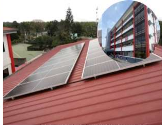
Five Storey Higher Education Building Capacity 20KVA
